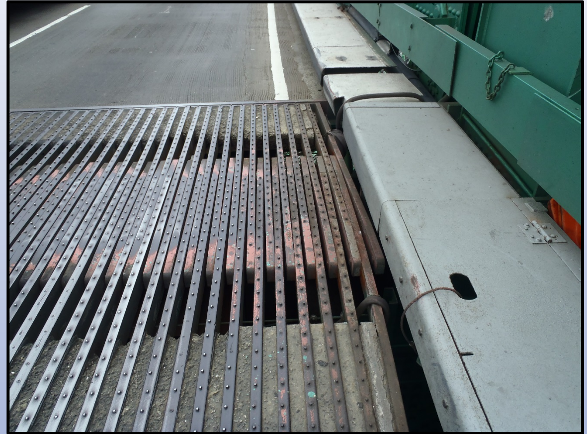
Large gap widths between the steel fingers.
