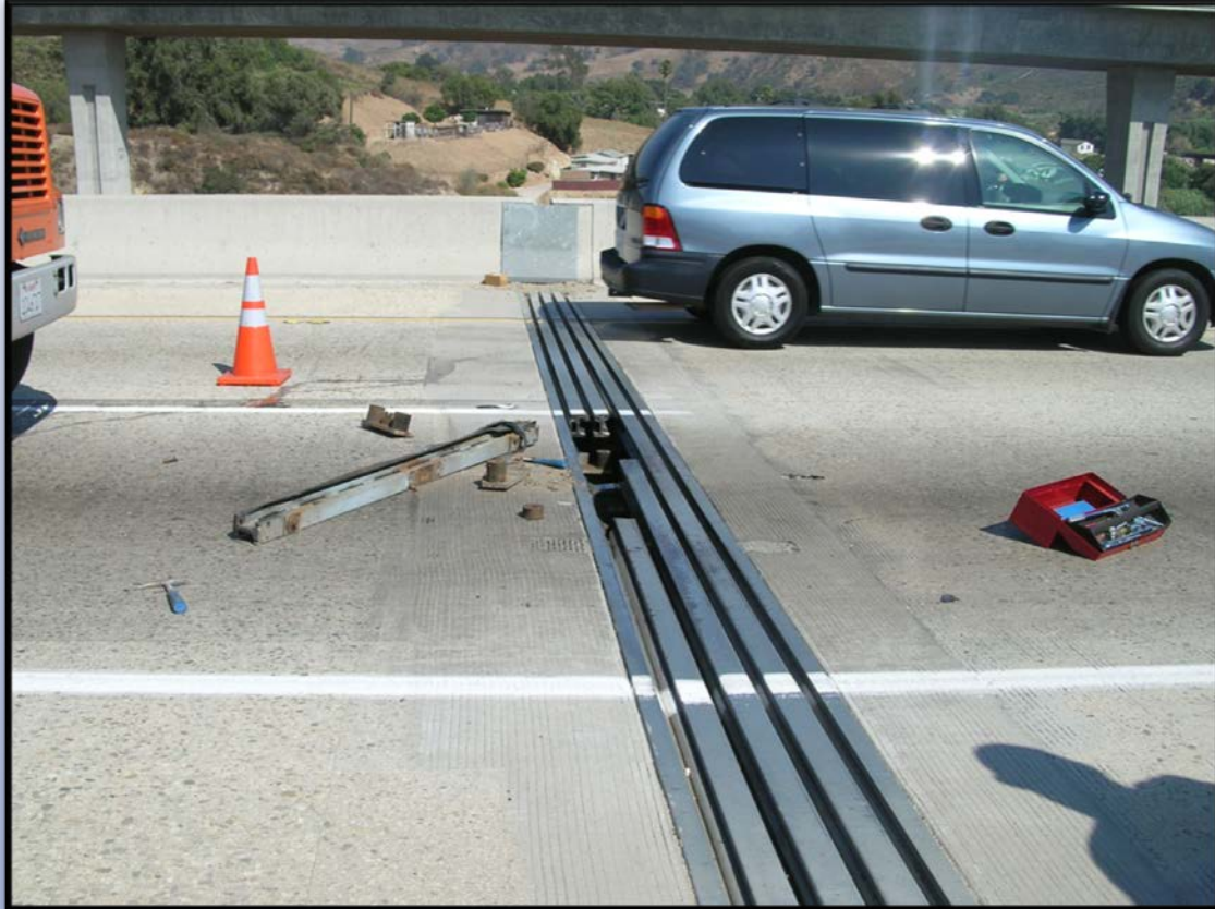
Broken center transverse beams.
