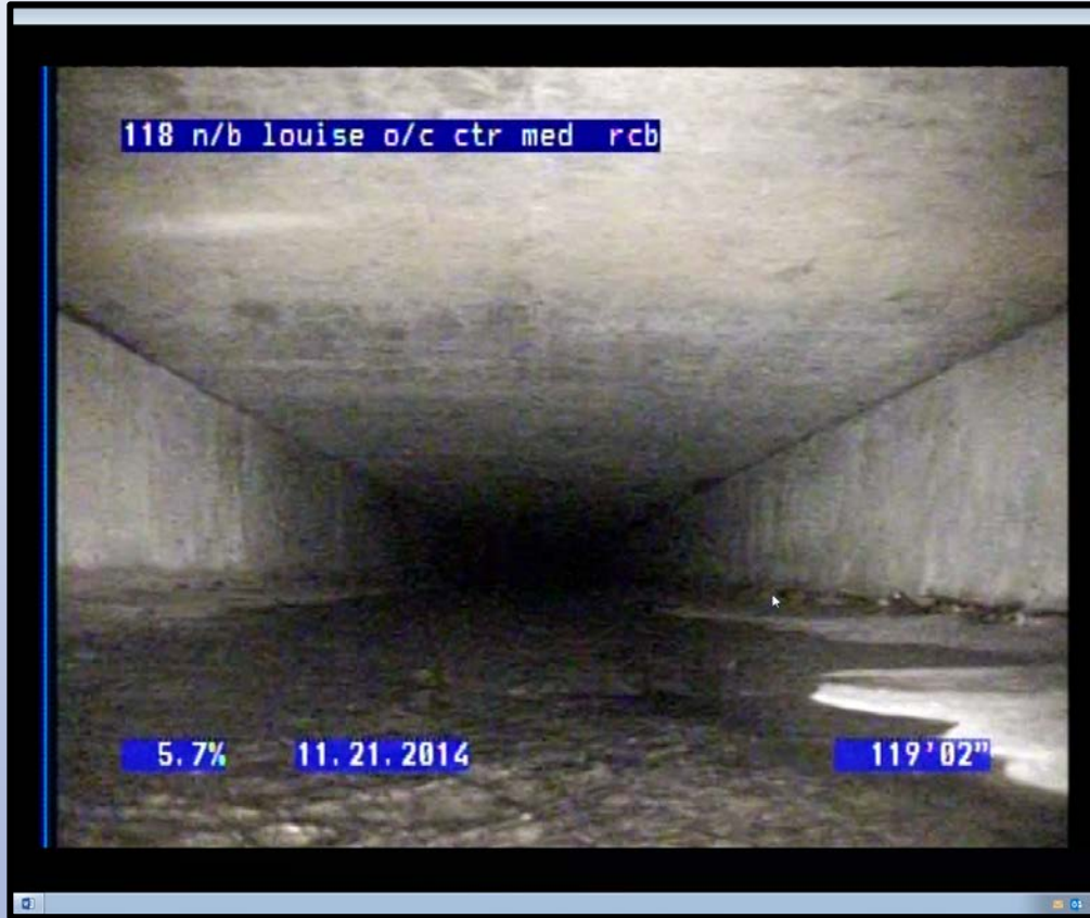
Confined Space (Robotic Inspection)
