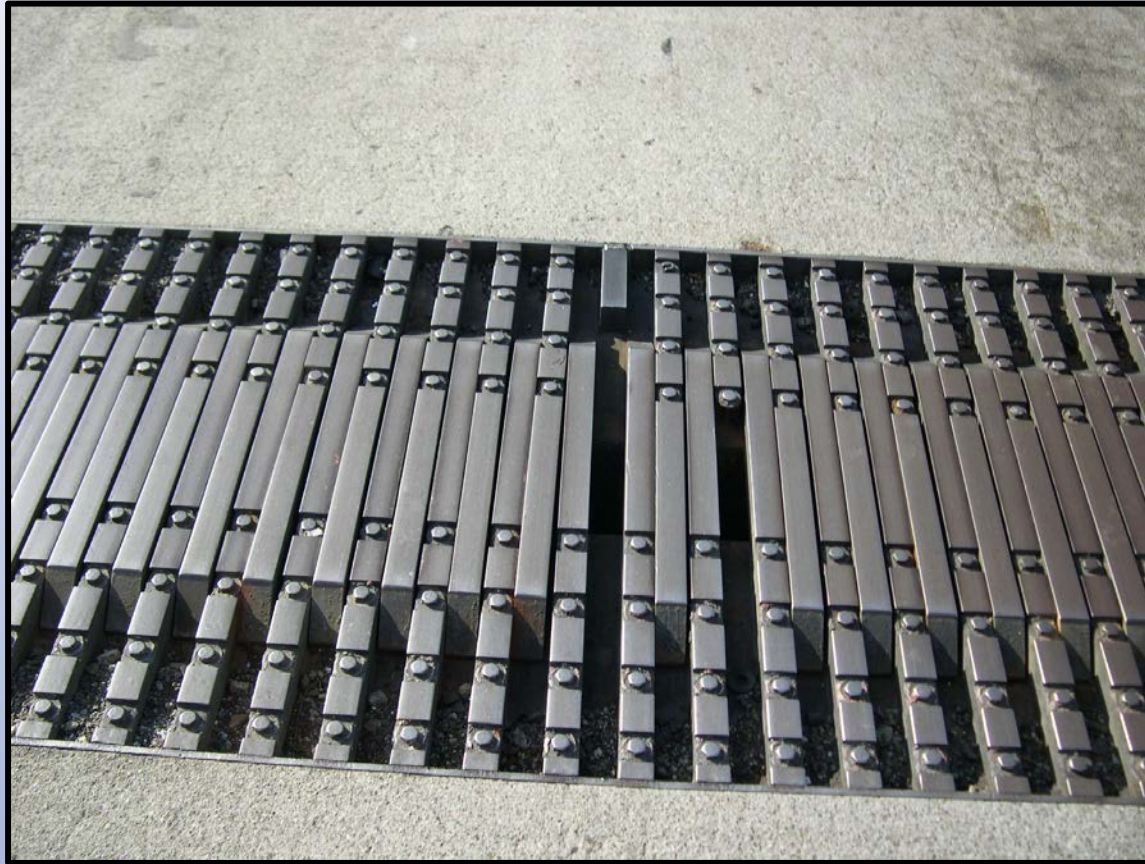
Breakage of the Steel Finger Elements.
