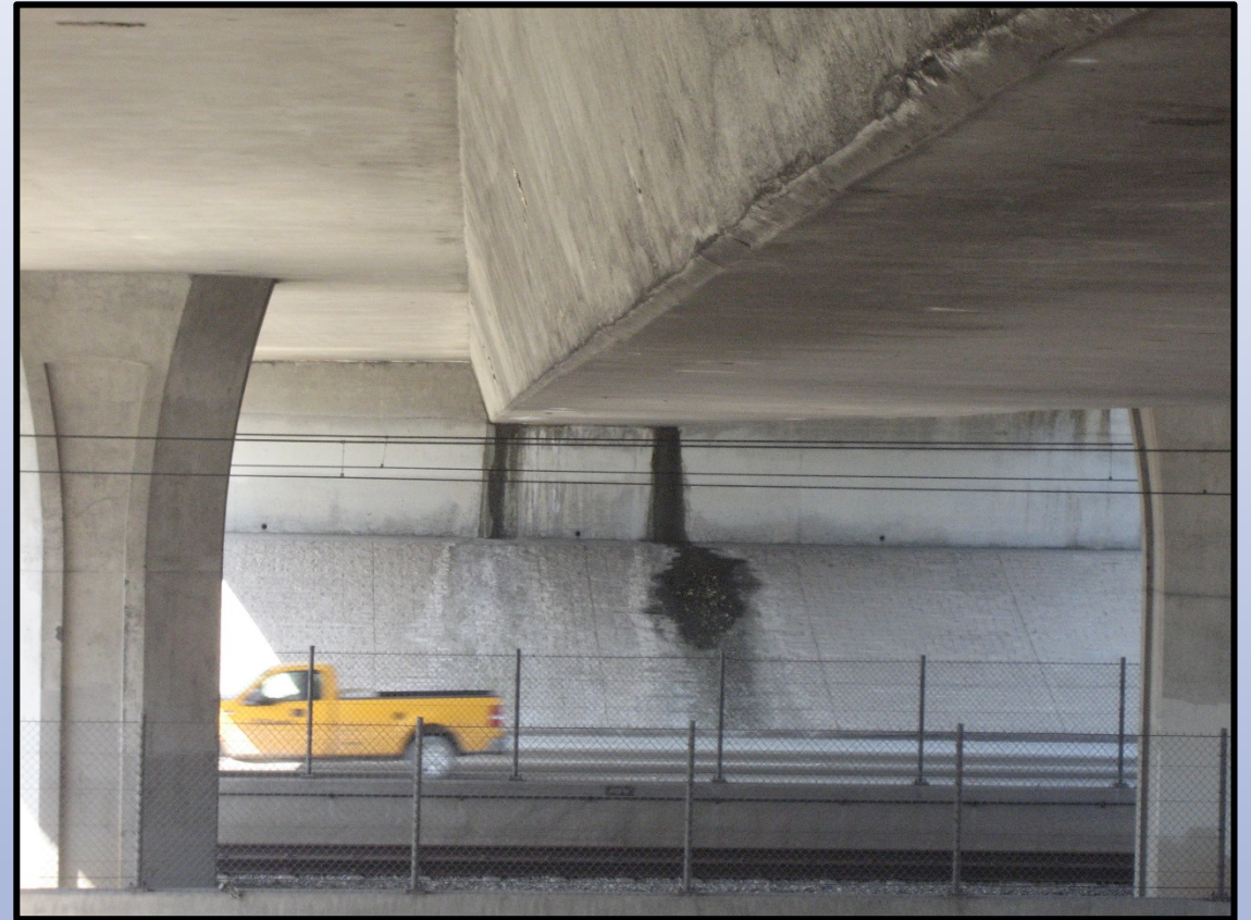
Failed and Leaking Joint Seal
