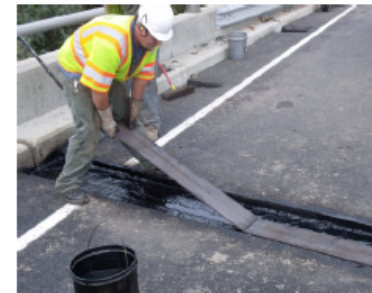
Figure 8.26 Bridging Plate Installation
