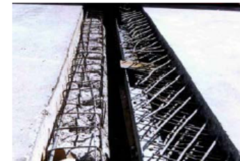
Figure A.21 Removed Joint System
