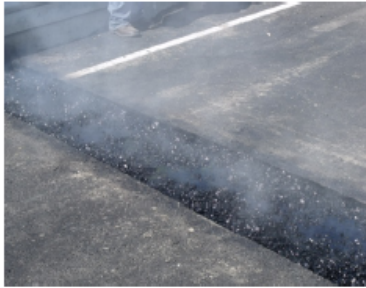
Figure 8.25 Plug Installation Showing Coated Aggregate and Binder
