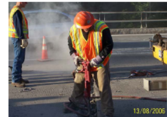
Figure A.20 Chipping out Concrete at Joint
