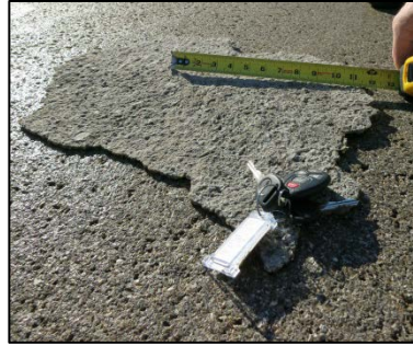
Thermal incompatibility, unsound substrate
