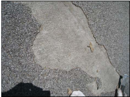
Visible concrete curing compound
