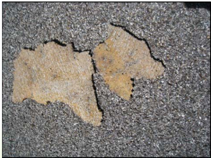
Visible contaminants, first course mixed off ratio
