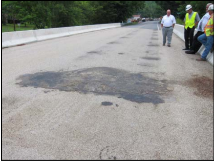
Improper mix ratio of the resin binder system
