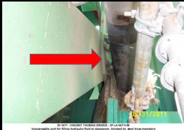
Viscous damper fill port blocked
