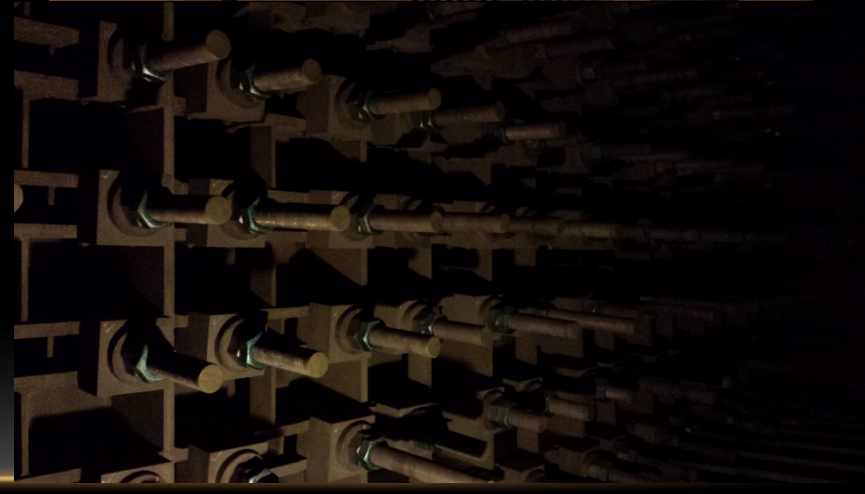
Lack of Internal Lighting
