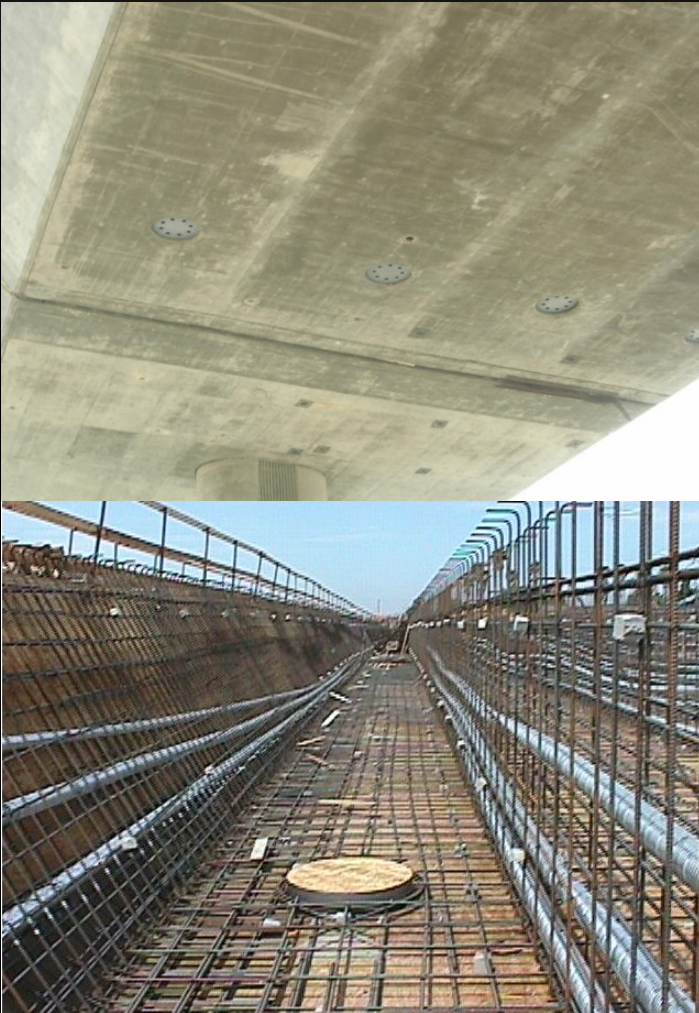
Box Girder Access
