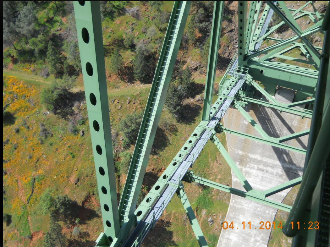
Fracture Critical Member Catwalk Inspection Access
