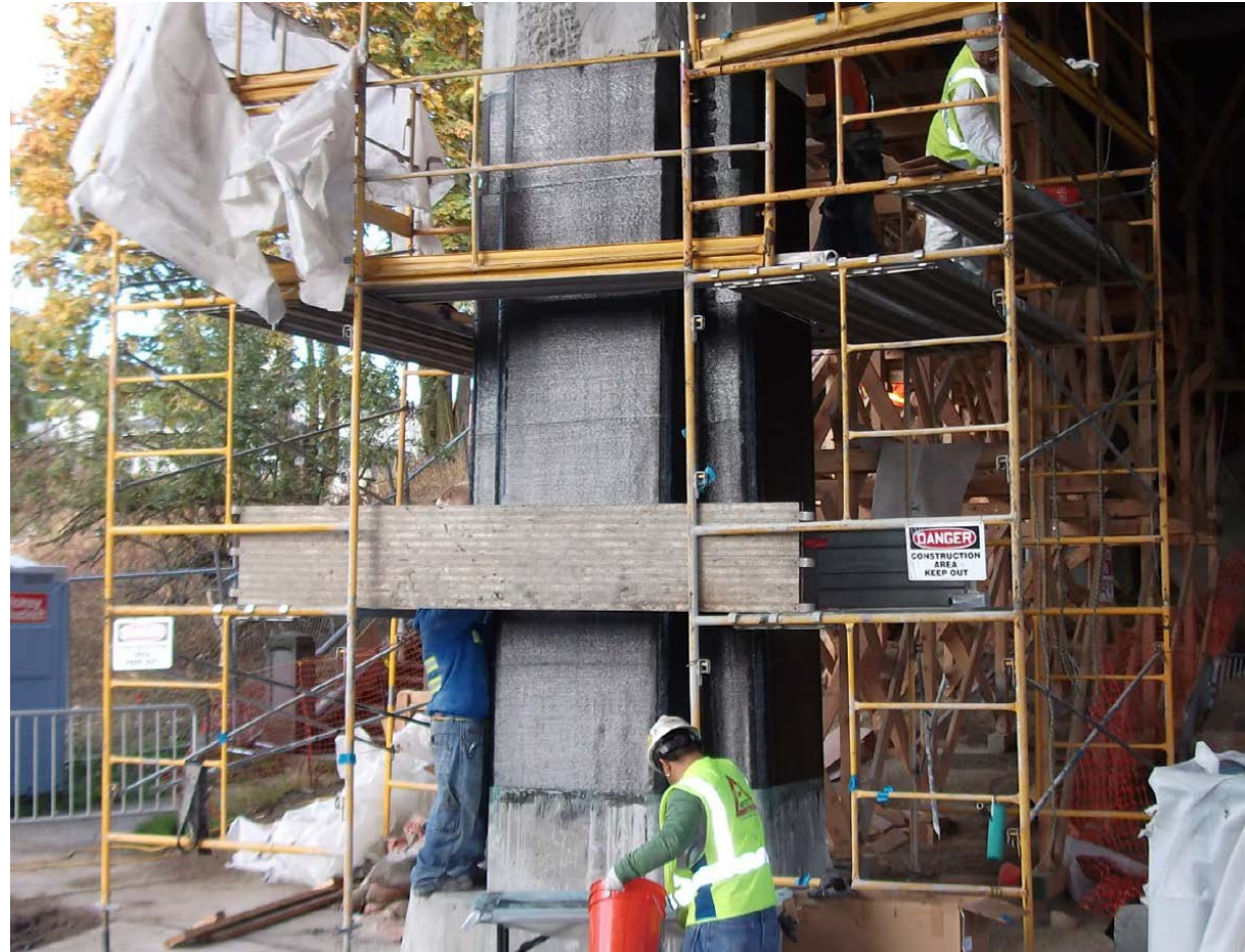
Seismic Retrofit Phase 3 (2011-12)
