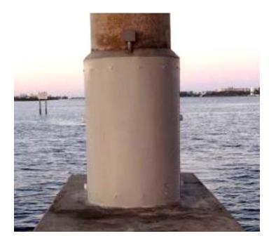
THE ZINC MESH ANODE IS PRE-INSTALLED INSIDE THE FORM TO PROVIDE AN ANNULAR SPACE OF 50+ mm WHICH IS LATER FILLED WITH MORTAR. SACRIFICIAL C.P. JACKET IS PLACED AROUND THE PILE AND CONNECTED DIRECTLY TO THE REINFORCEMENT WITHOUT AN EXTERNAL POWER SUPPLY.
