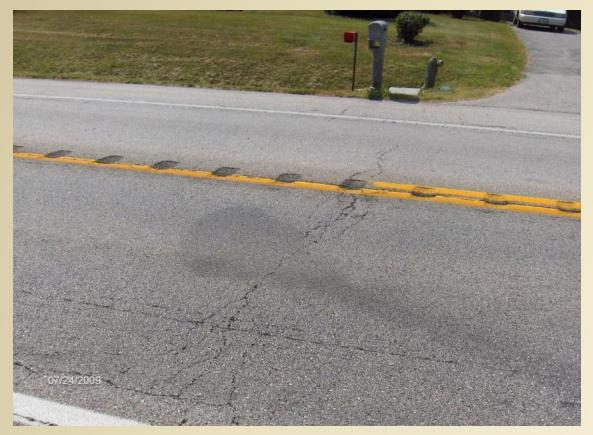
Composite Pavement – PCC joints reflect through HMA.
