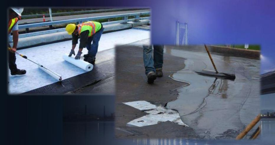
Reinforcing fabric is embedded into the membrane while it is still warm and tacky.
