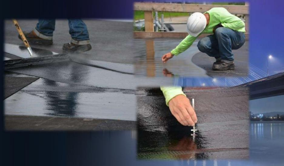
Membrane should be 215 mils (5 mm) thick
