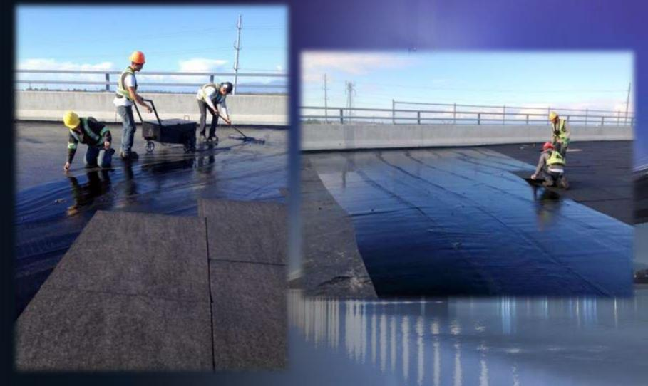
Membrane should be 215 mils (5 mm) thick
