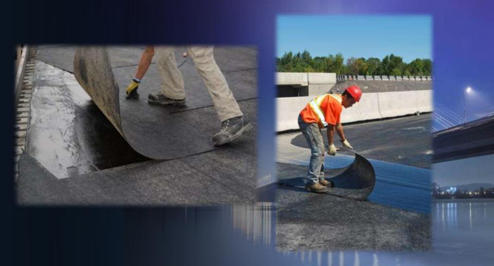
Install the protection board in a staggered pattern – 1" overlap
