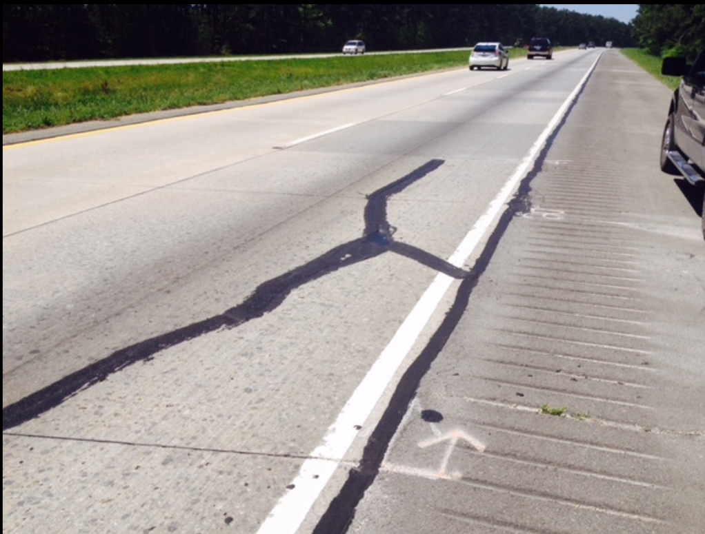
Center slab Crack Repair Rt 20 - GA
