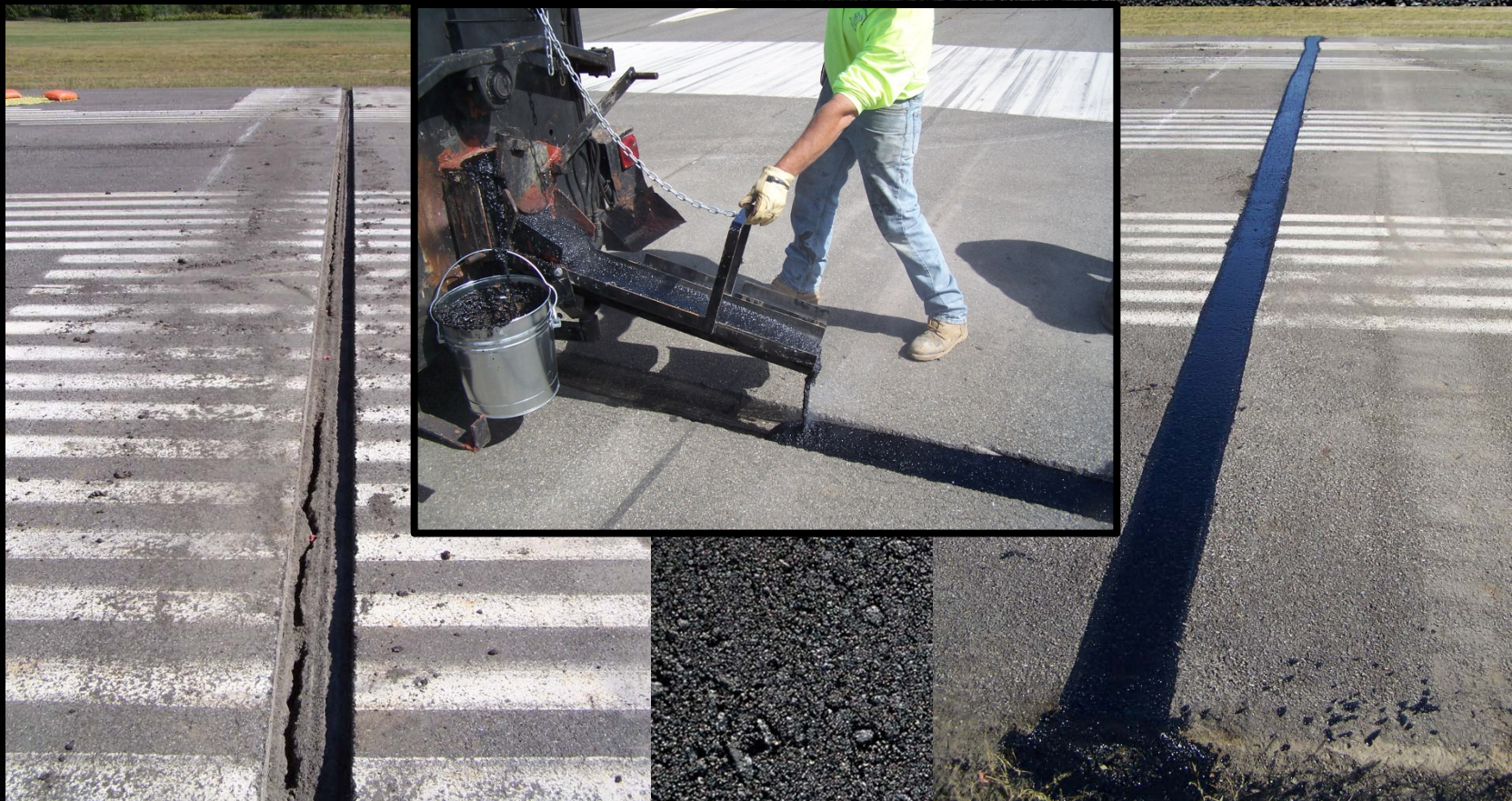
GA Airport Transverse Crack Repair – Lake Placid, NY –
