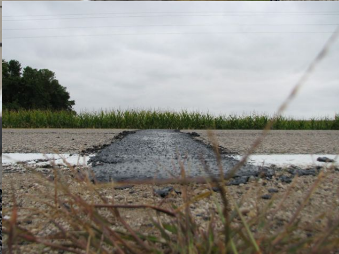
Repair of Cupped Joints- Minnesota
