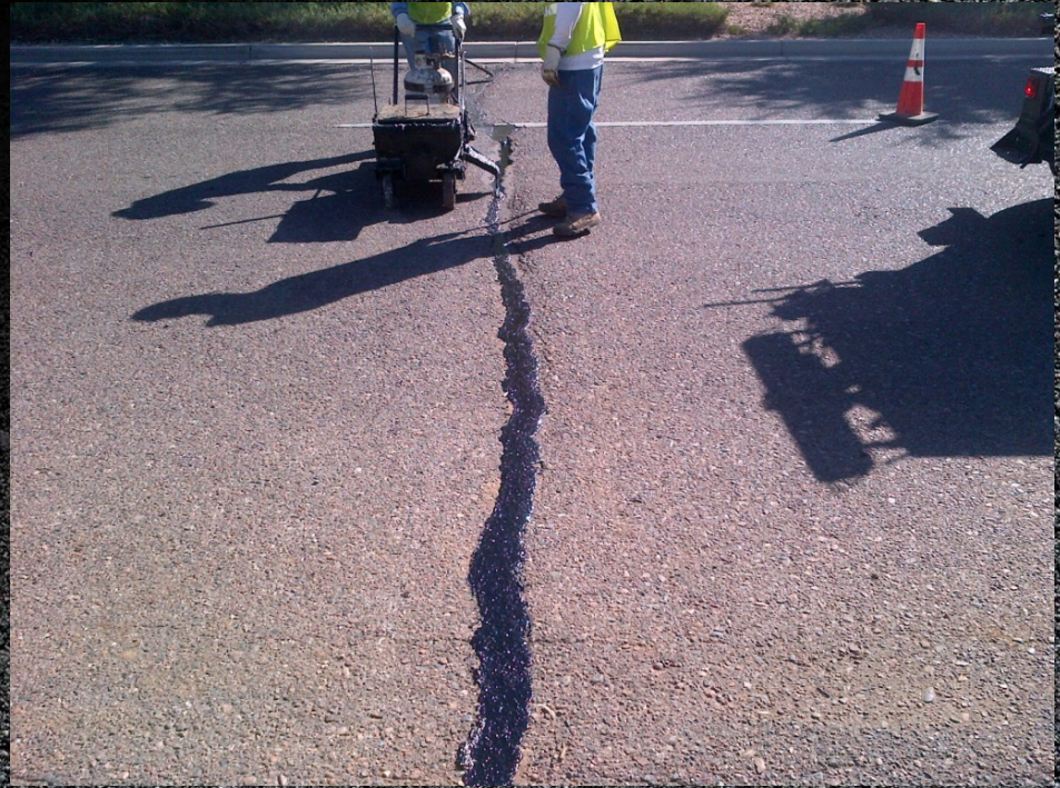
Large Crack Repair Phoenix, AZ
