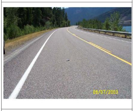
Condition: Cover Material Loss Attributed to Insufficient Embedment Caused From Plant Mix Surfacing Segregation.
