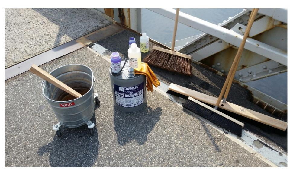
High Molecular Weight Methacrylate Crack/Surface Sealer
