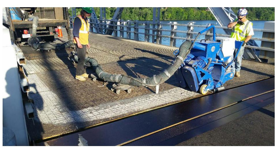
Shot Blast Excess Cured Sealer on Deck Surface For Application of Epoxy Overlay
