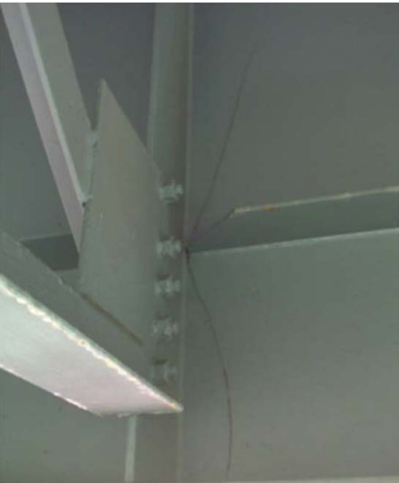
2012 Fractures on N.B. and S.B. Bridges
