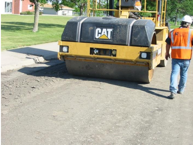
Final compaction (often in combo with pneumatic)
