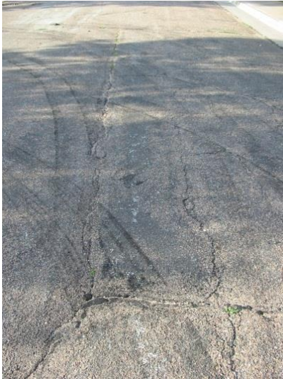
Road before pulverization
