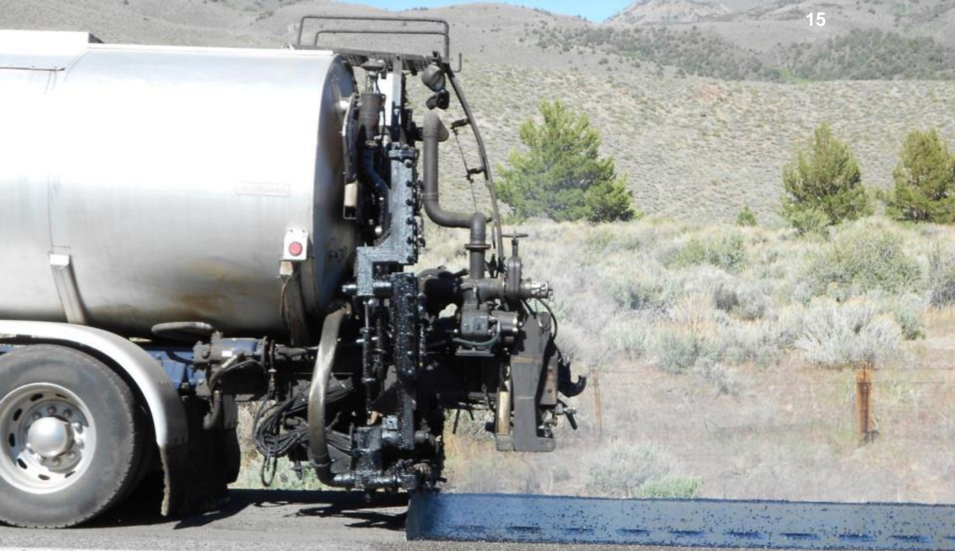
Mainline AR Gap Grade Shoulders 70-10 dense grade
