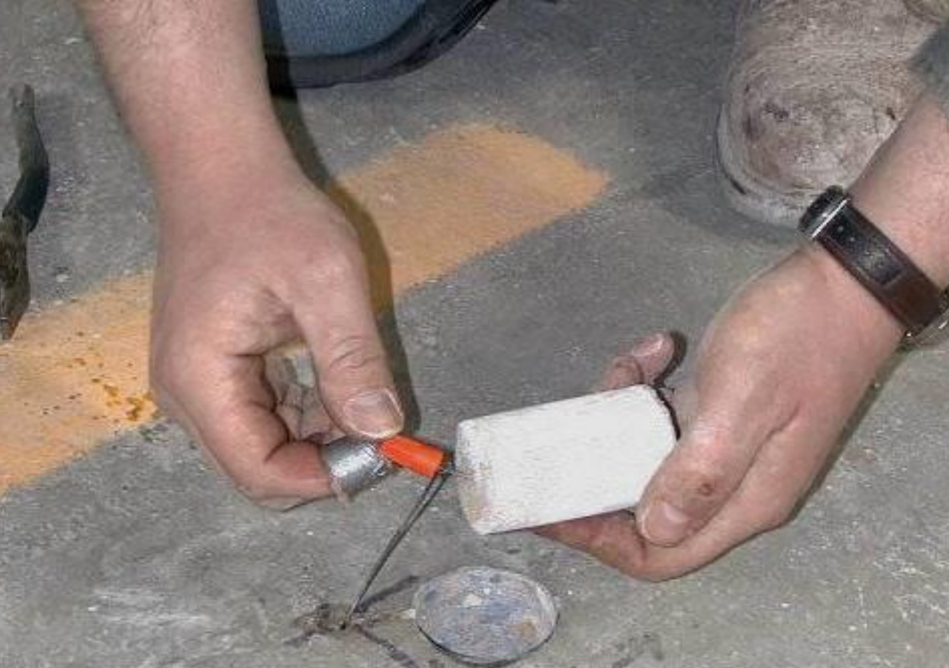
Anode Connection to Reinforcing Steel
