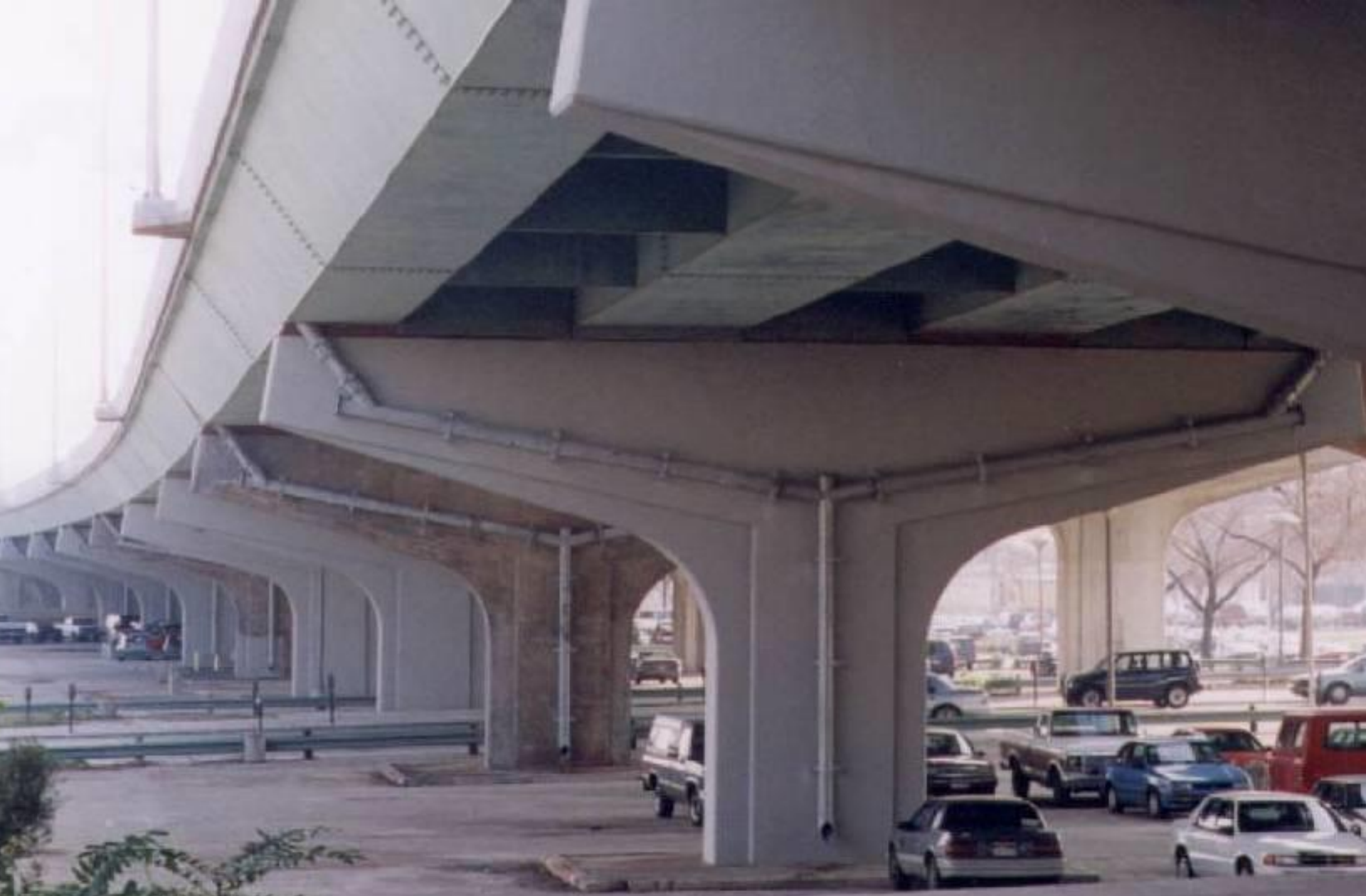
Piers after ECE Treatment Cleaned and Sealed
