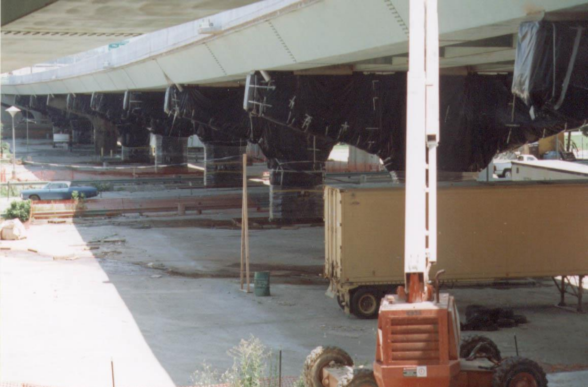
Several Piers Wrapped and Undergoing ECE Treatment Omaha, Nebraska
