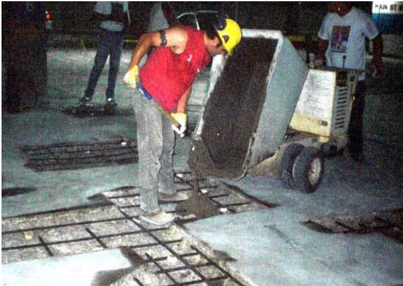
Embedding anodes with repair material.
