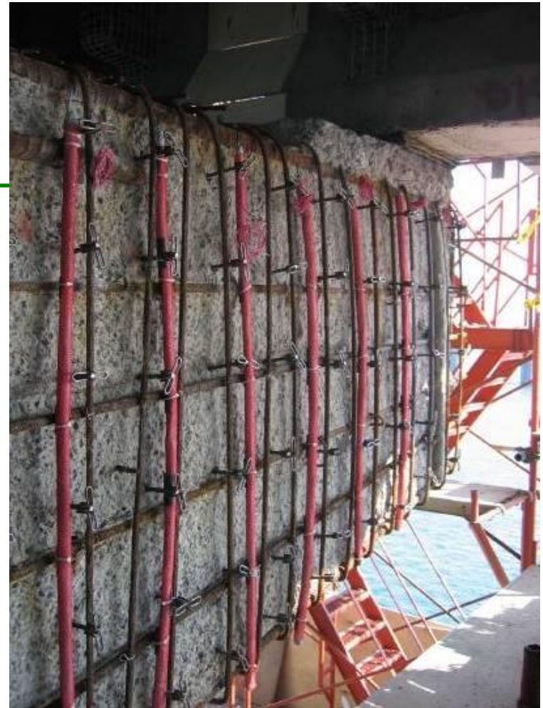
Bridge Pier Cap Repair with Galvanic Anode Strips
