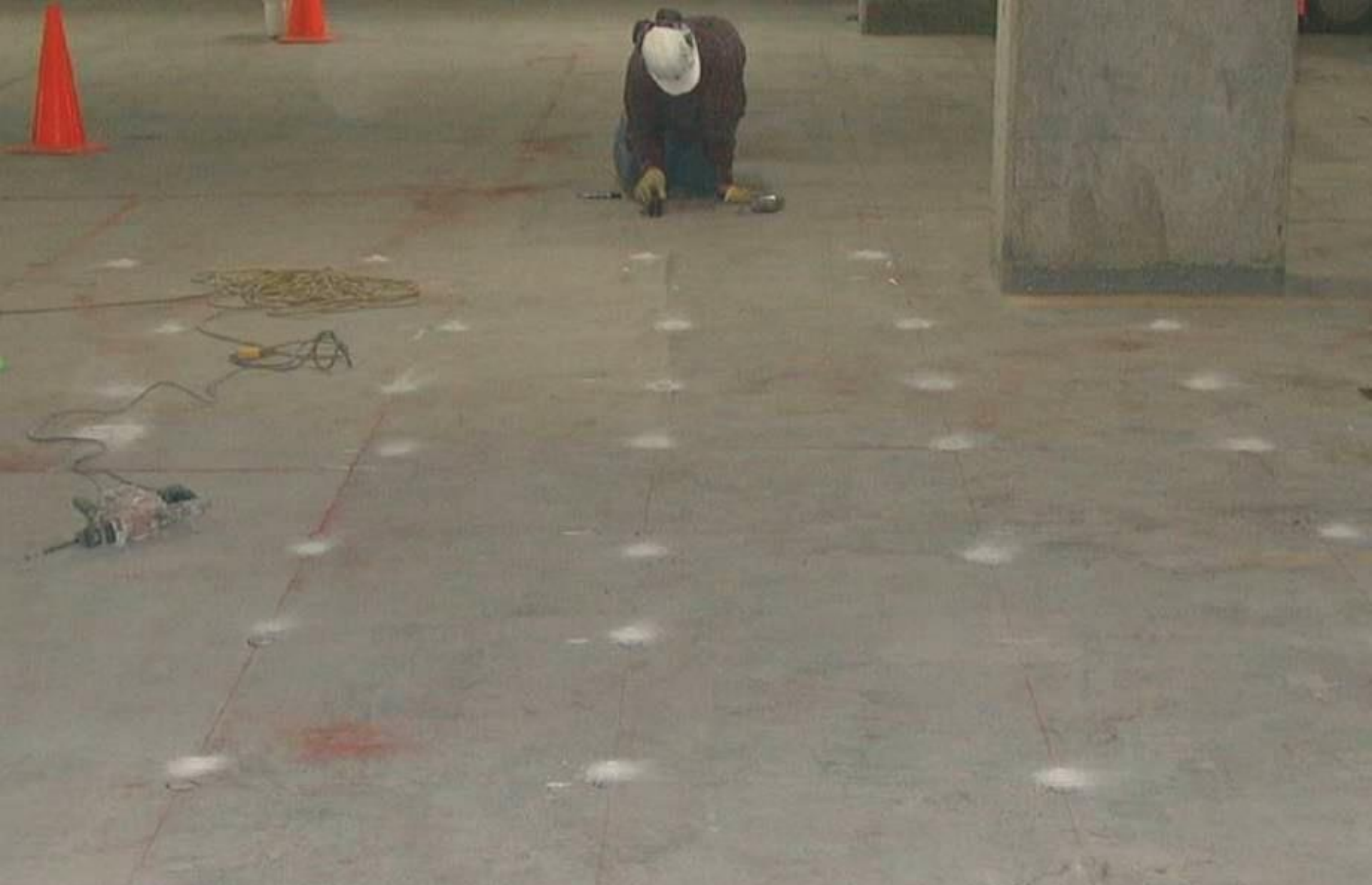
Predrilled Holes for CC Installation Parking Garage Deck
