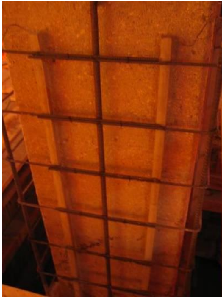
Bridge Column Repair with Reinforced Concrete Jacket
