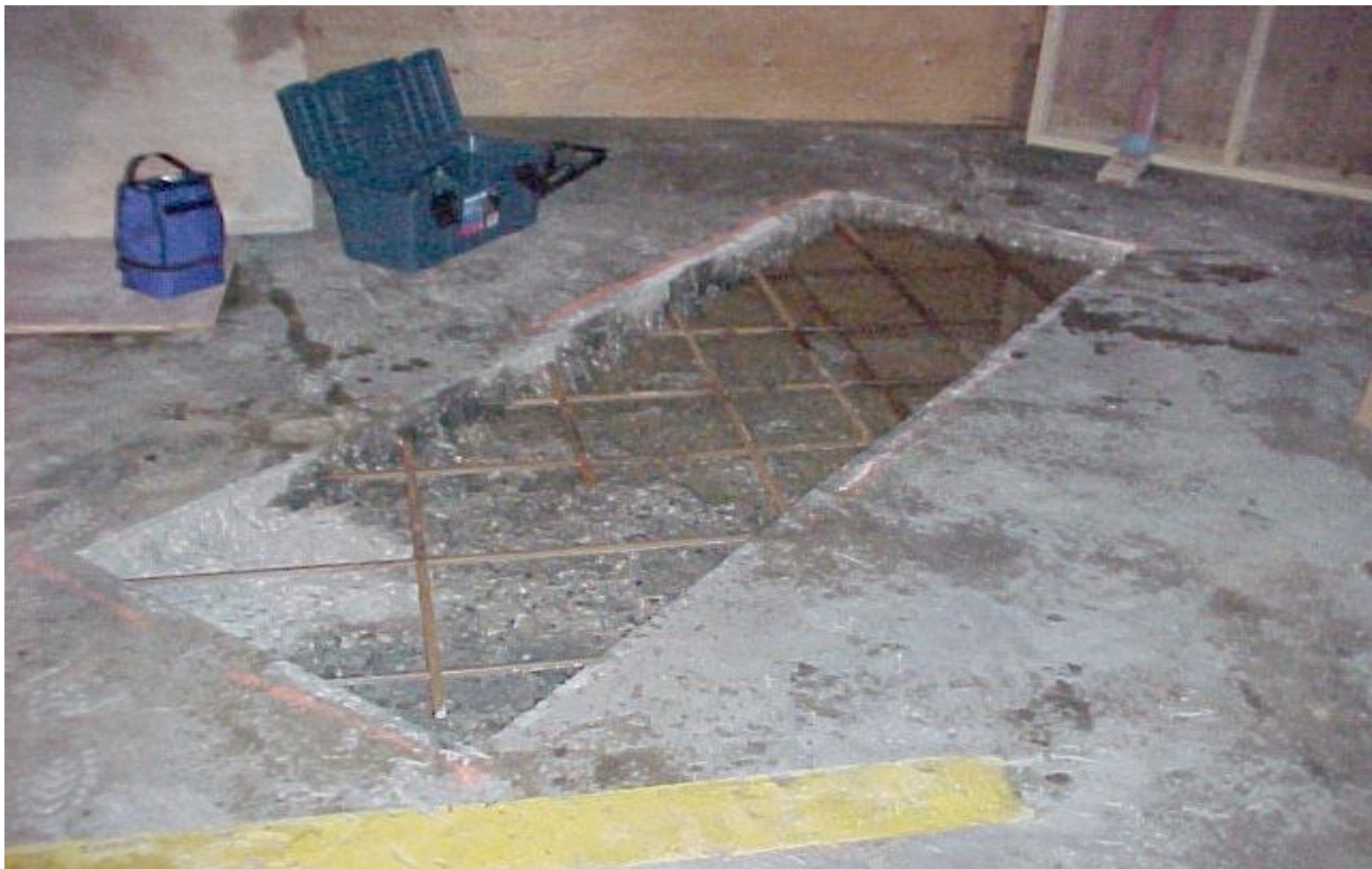
Saw cut and cleaned repair area.
