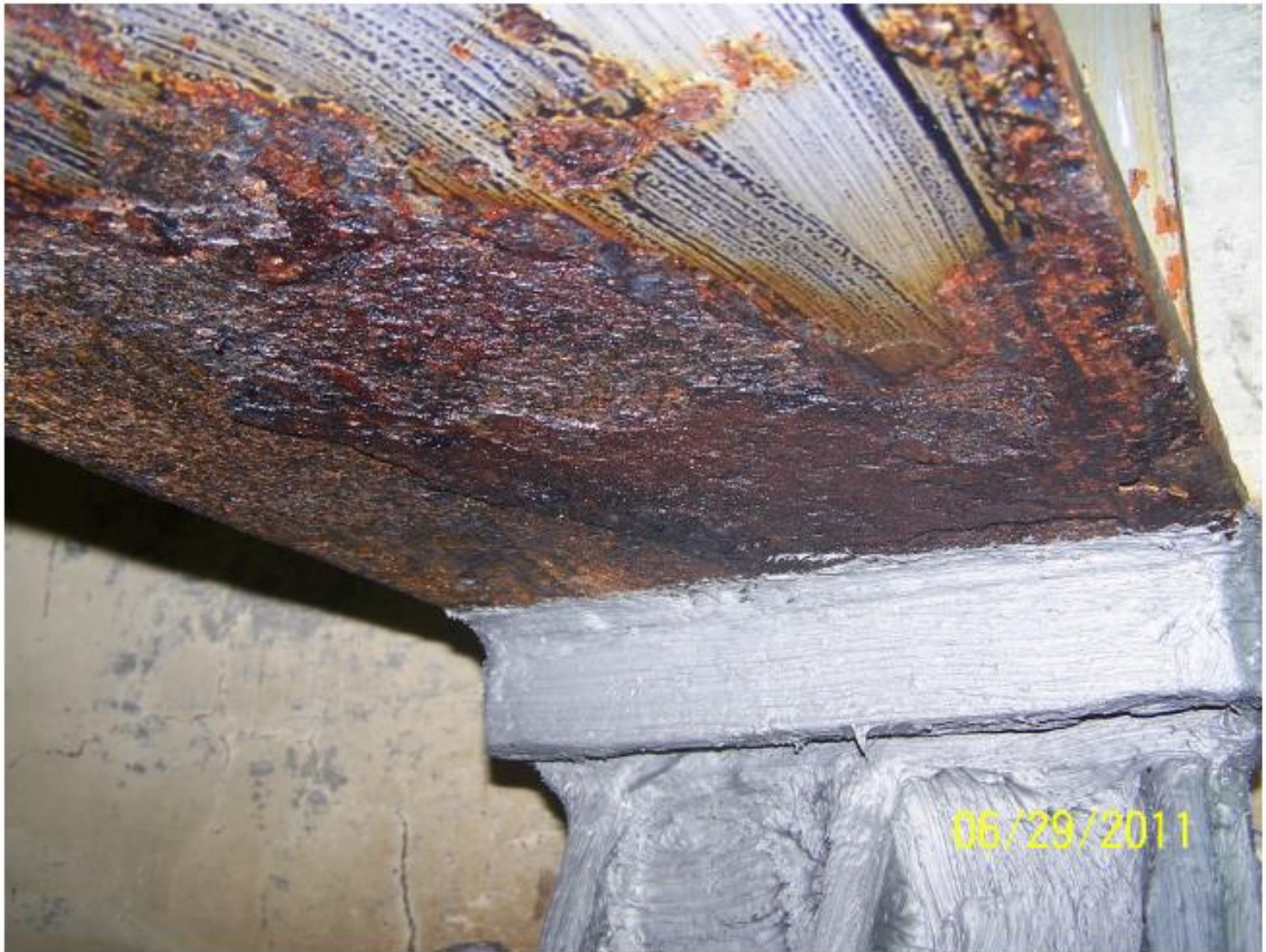
Pic of the black-max and grease application
