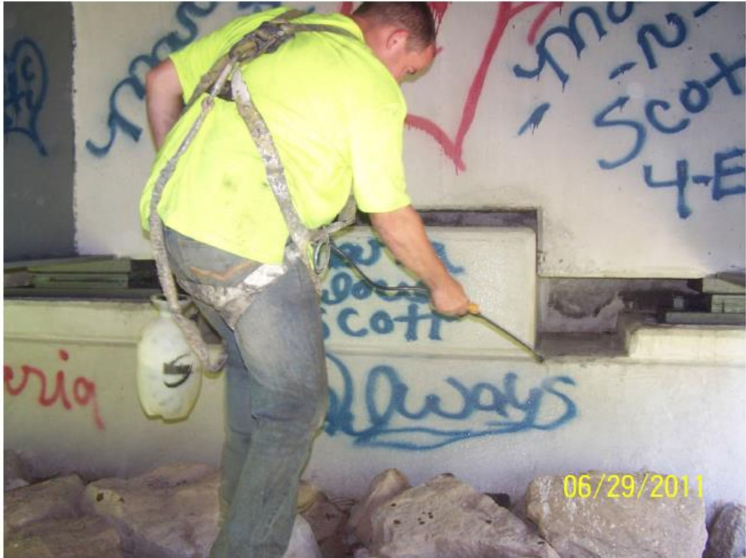
Example application of Clear Cladding concrete sealer
