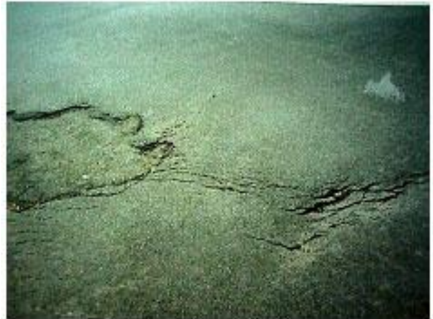
Slippage/Shear Cracks
