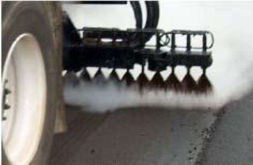
Proper Spraying - Even
