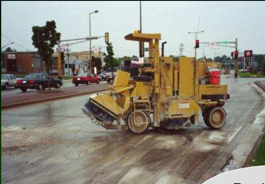
Partial Depth Patching
