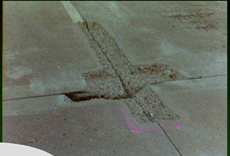
Partial Depth Patching
