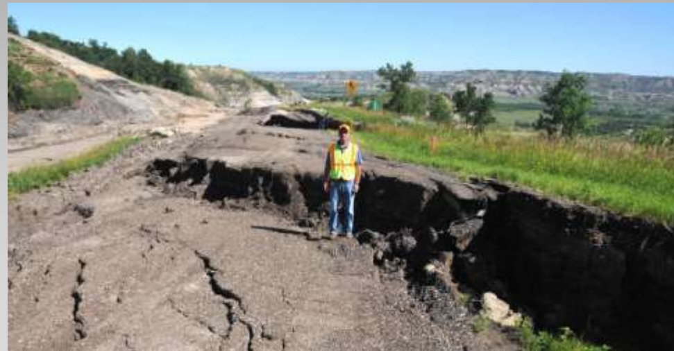
Dickinson District Engineer Larry Gangl stands in landslide area on ND Highway 22 north of Killdeer – July 2011.
