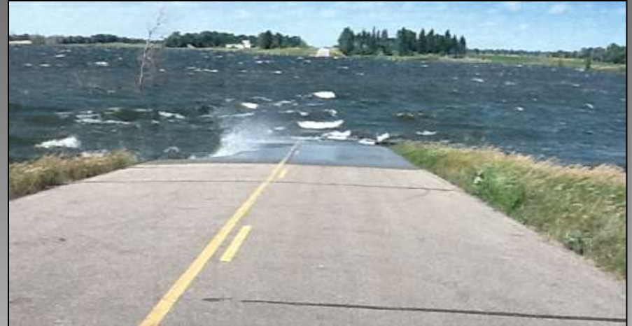
Lamoure County roadway
