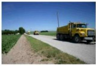
a) The triple shot bituminous surface treatment and crushed gravel course shall be constructed under the direction of the Public Works Department and shall consist of an application of penetration asphalt followed by two applications of crushed gravel seal coats. The Public Works Department must check all applications.
