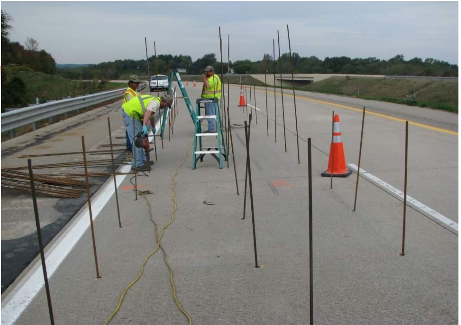
Slab jacking on M-6 near Grand Rapids
