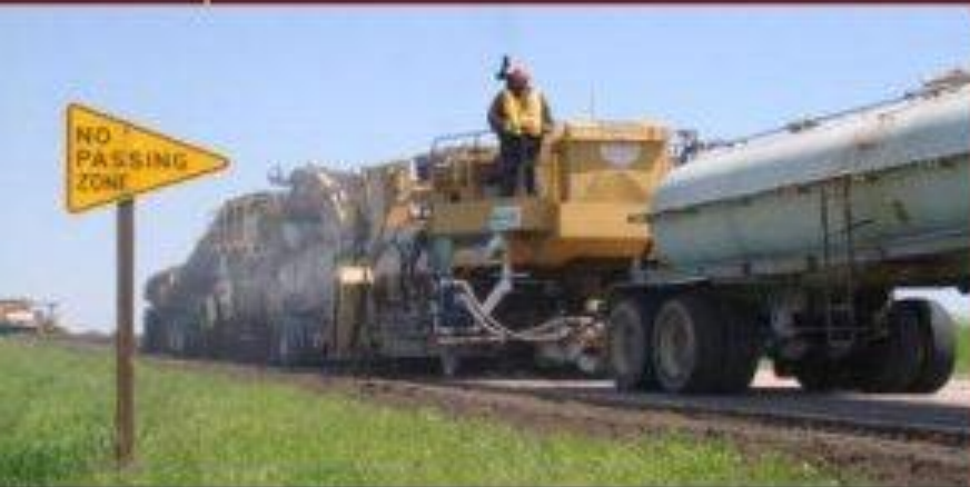
Hydrated Lime Slurry Stabilization
