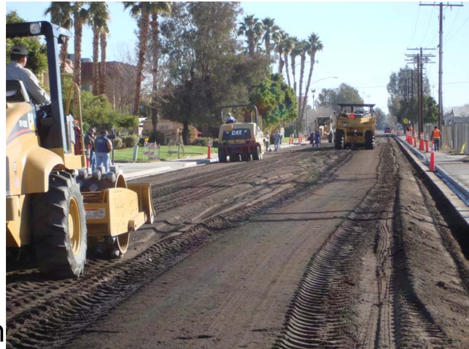
City of El Centro, CA 2008 FDR Project
