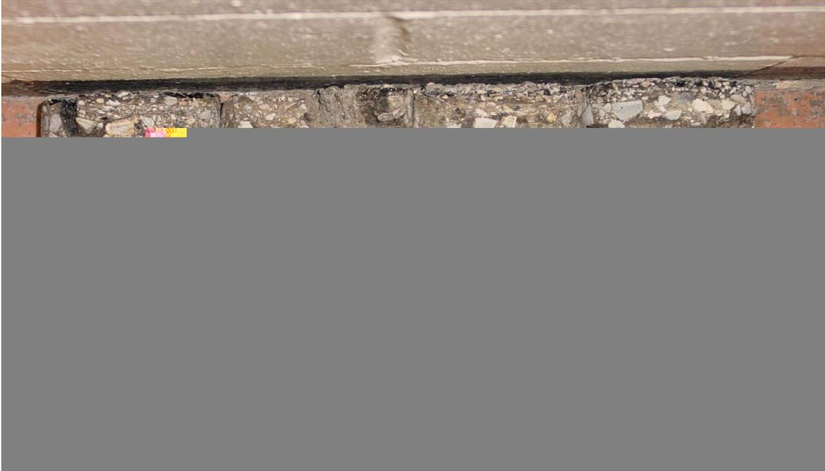
Before Construction: Light to Heavy Stripping, Delaminated, and Fell Apart
