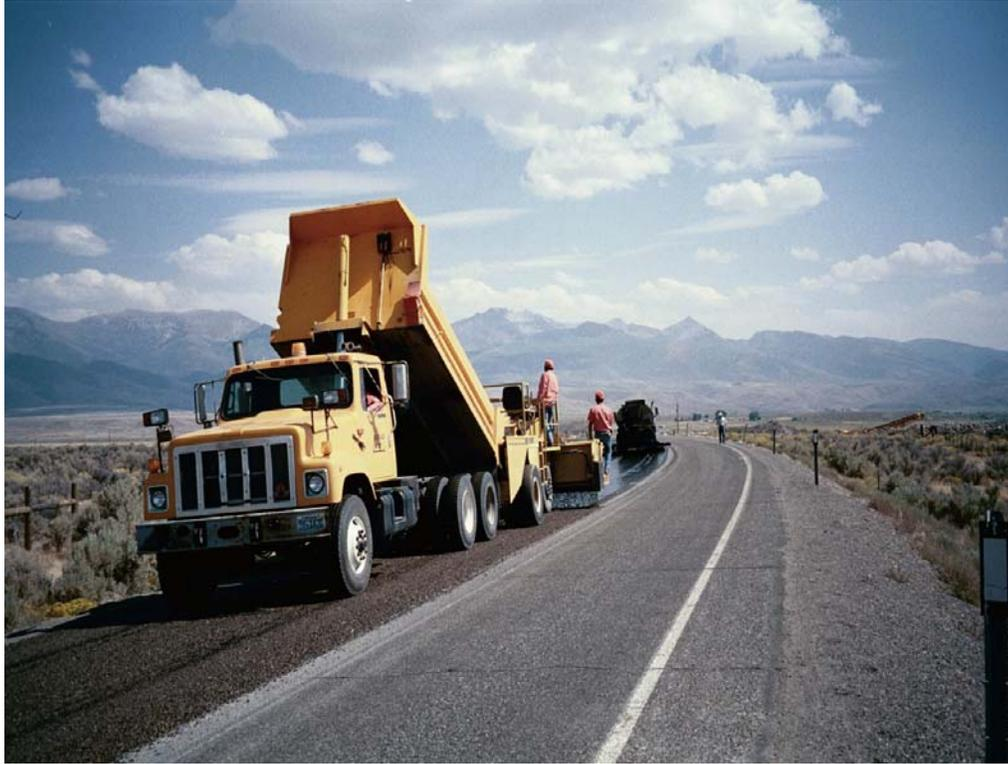
**FIGURE 5.1b Maintenance personnel place chip seal.**
