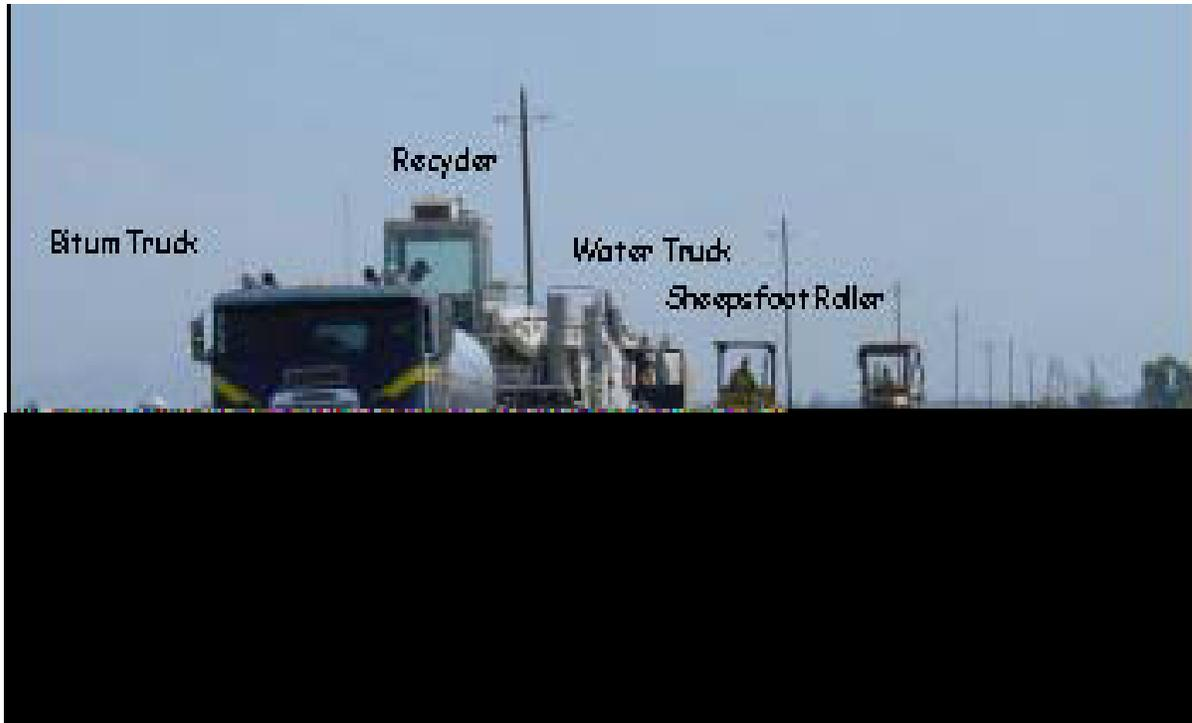
**FIGURE 2.6b Example of typical foamed asphalt equipment (3).**
