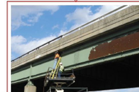
Lincoln Tunnel Interchange, NJTA
