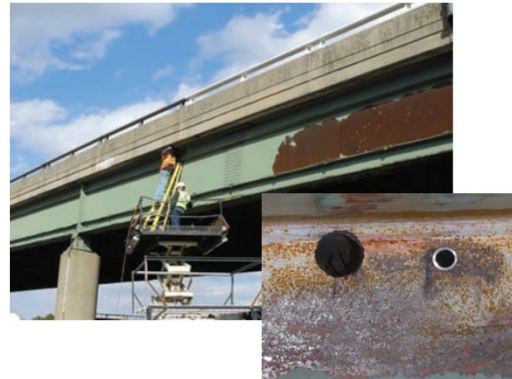
Lincoln Tunnel Interchange, NJTA (Mar 2012)
