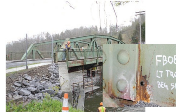
Bridge over Delaware River, NYSDOT (Apr 2012)
