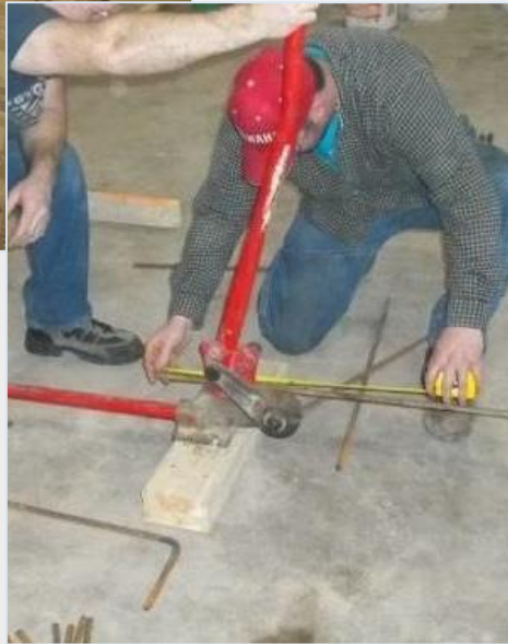
Cut, Bend and Place Reinforcing Steel
