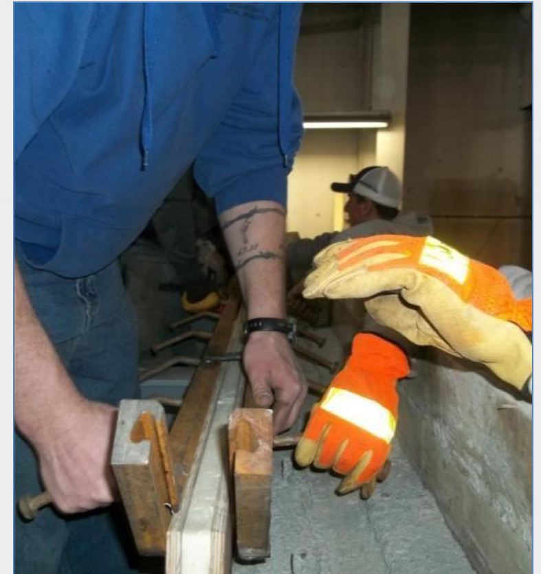
Install Strip Seal Extrusion
