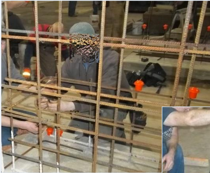
Cut, Bend and Place Reinforcing Steel
