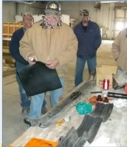
Strip Seal Gland Repair Demonstration
