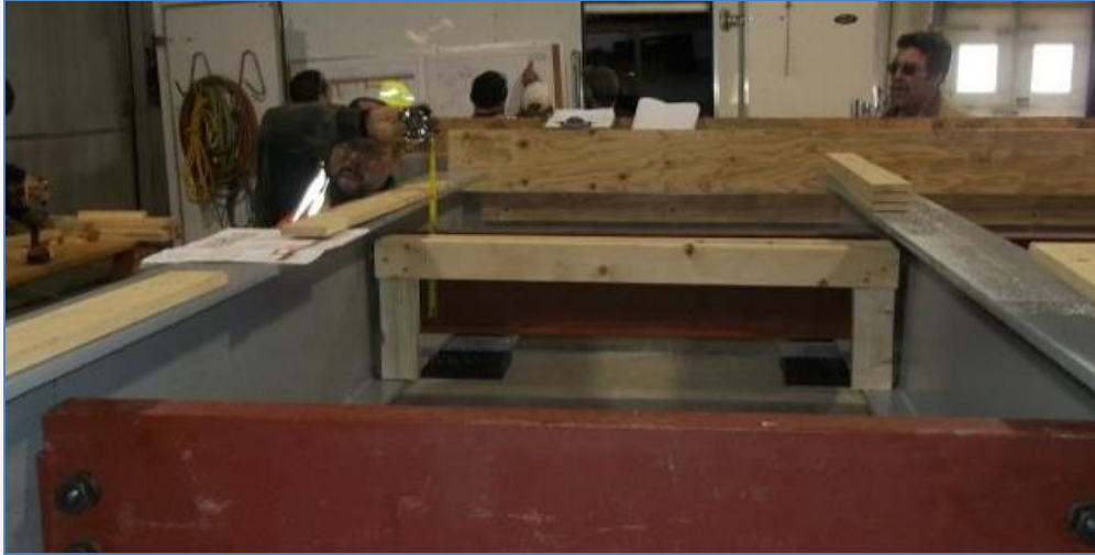
Construct Deck Falsework
