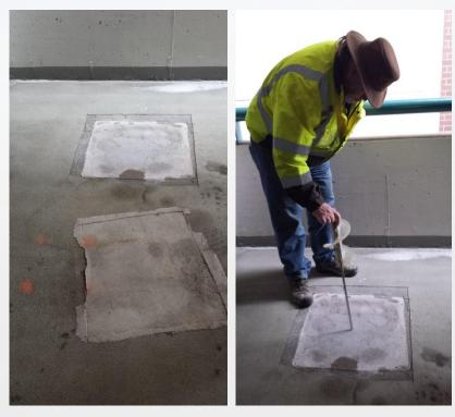
**Square patch:** No cracks. No debonding (sound test with a rod).
