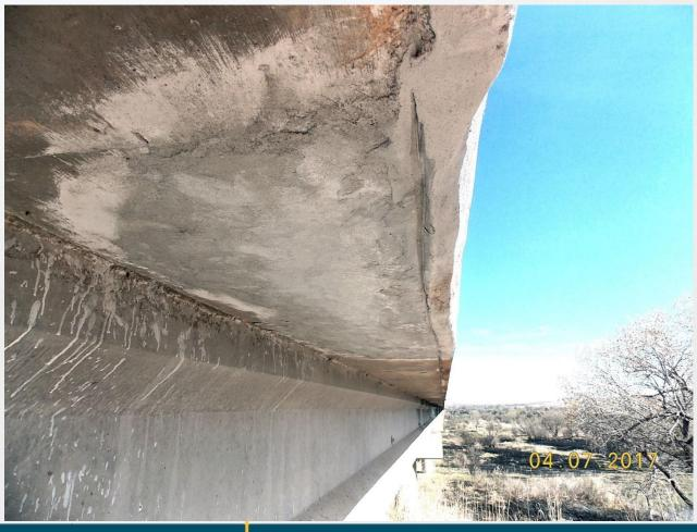
Anode will form at the lower pH region which in this case is at the repair material.
