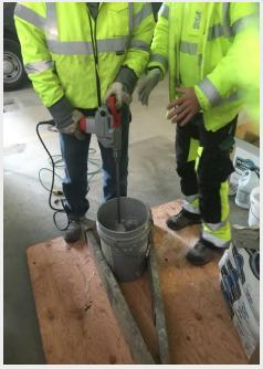
Trapezoid Patch: 2 x 2 ft. - 4 in. deep. Square Patch: 2 x 2 ft. - 3 in. deep Saw cut edges. Dry concrete. CSP = 5. Clean rebars. 45 sec. mixing time per batch with an electric drill with auger.
