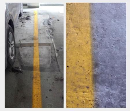
**Trapezoid patch**: Hairline crack at the center of the patch. Approx. 3 inch long. No debonding.
