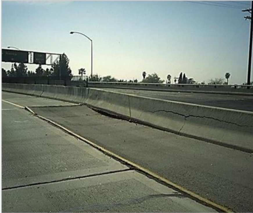
Figure 62: Approach slab settlement and cracking of the concrete barrier ( NISEE )
