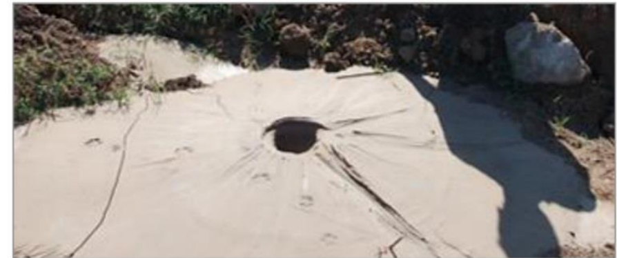
Figure 102: Liquefaction sand boil
