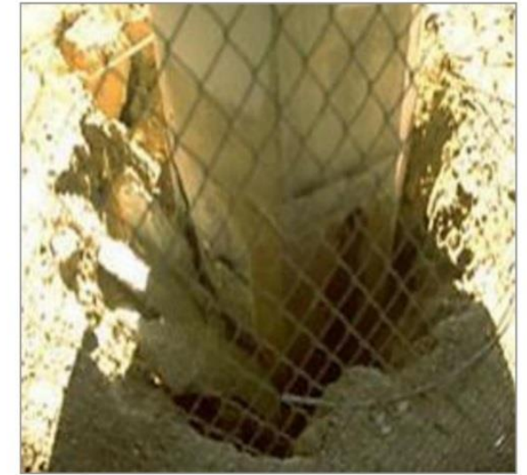
Figure 100: Ground movement indicating possible foundation problems ( INDOT )
