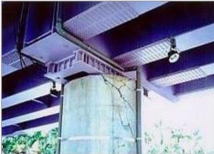
Figure 95: Compression failure on the top of concrete bridge pier ( INDOT )
