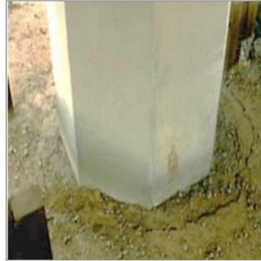
Figure 100: Ground movement indicating possible foundation problems ( INDOT )
