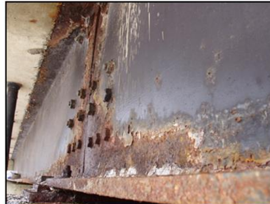
Element: Fascia Beams (View B) Condition State: 4 (Severe) >16% corrosion/defects
