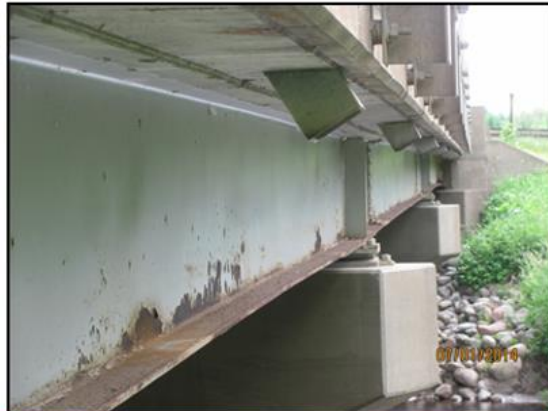
Element: Fascia Beams (View A) Condition State: 4 (Severe) >16% corrosion/defects
