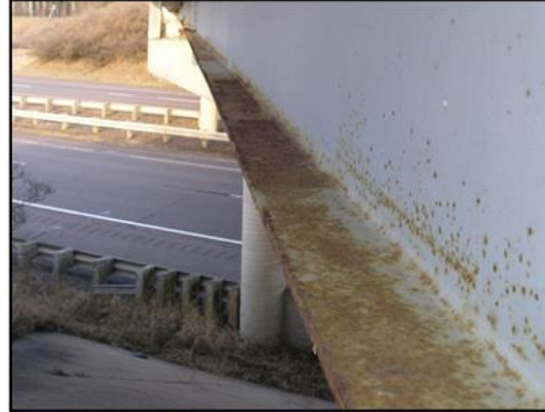
Element: Fascia Beams (View B) Condition State: 3 (Poor) >3 – 16% corrosion/defects
