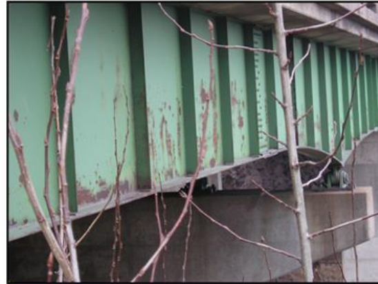
Element: Fascia Beams (View A) Condition State: 3 (Poor) >3 – 16% corrosion/defects
