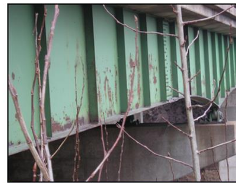
Element: Fascia Beams (View A) Condition State: 3 (Poor) >3 – 16% corrosion/defects
