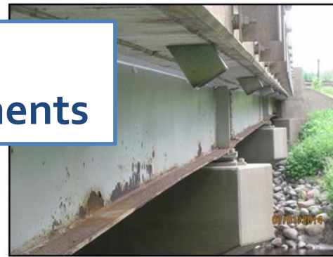
Element: Fascia Beams (View A) Condition State: 4 (Severe) >16% corrosion/defects
