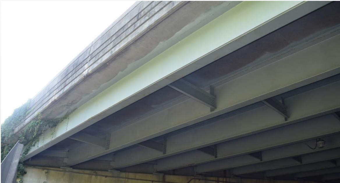
Bridge 1186: I-84 over Starr Ave.
