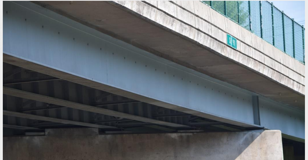
Bridge 1199: SR911 over I-84
