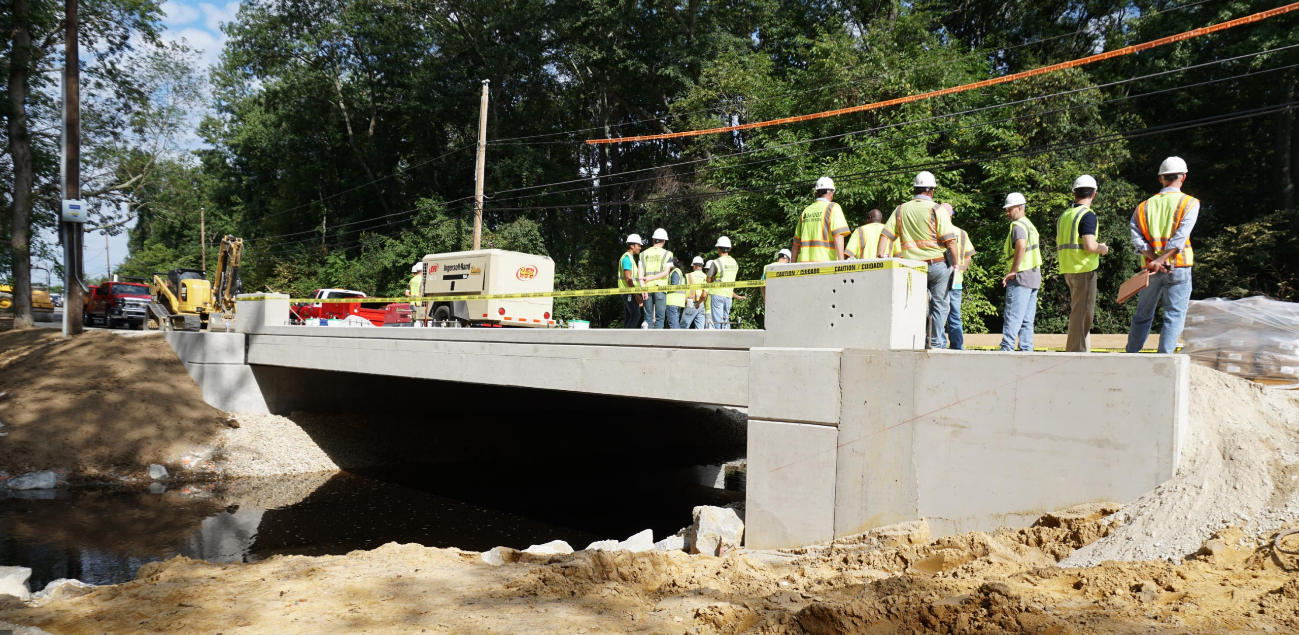
BLACKBIRD CREEK BRIDGE, DELAWARE
