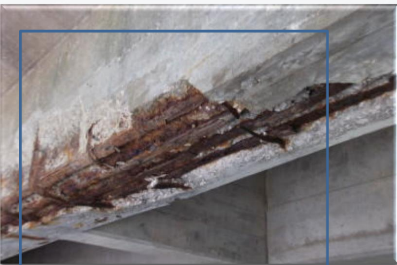
Severe Spalling
