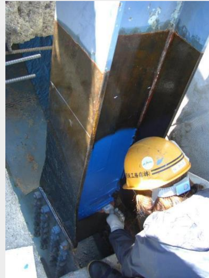
UHM CFRP Strand Sheets used to restore lost cross-section
