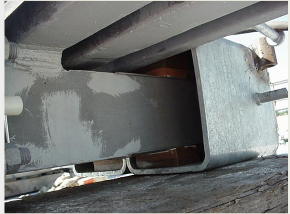
Pre-installation photo underneath modular expansion joint
