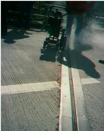
Saw cut to the limits of the new header.
