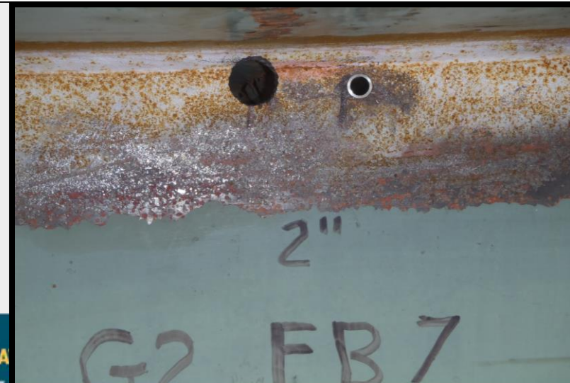
Repair Complete: 'Crack Arrest Hole' (left), 'StopCrackEX Hole' (right).
