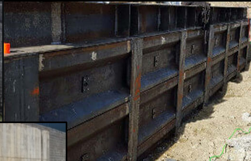
Steel Sheet Bridge Repair Washakie County, WY
