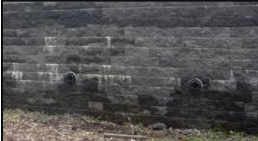
Block Wall Stabilization Pottstown, PA
