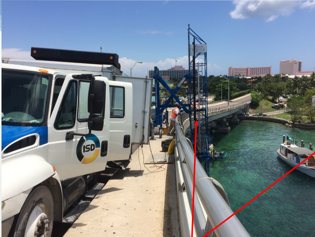
Hydra Platform for beam repairs under deck
