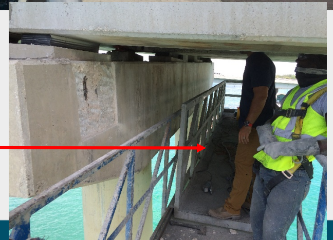
Hydra Platform for beam repairs under deck
