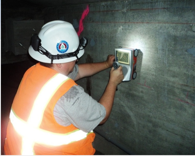
GPR to Locate PT Duct
