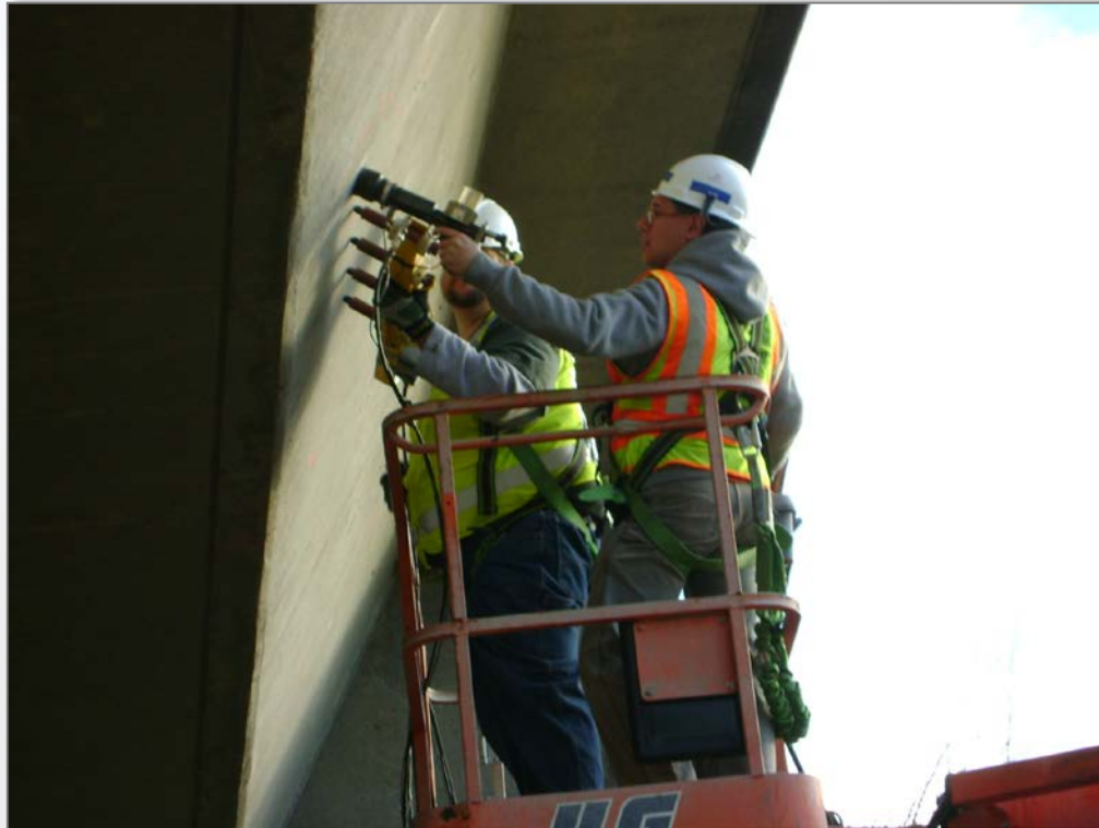
Internal PT Ducts
