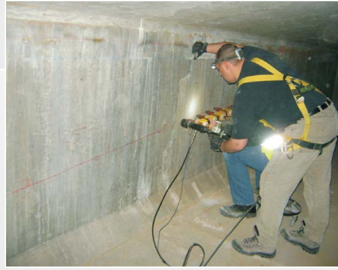
Impact-Echo Testing for Voids
