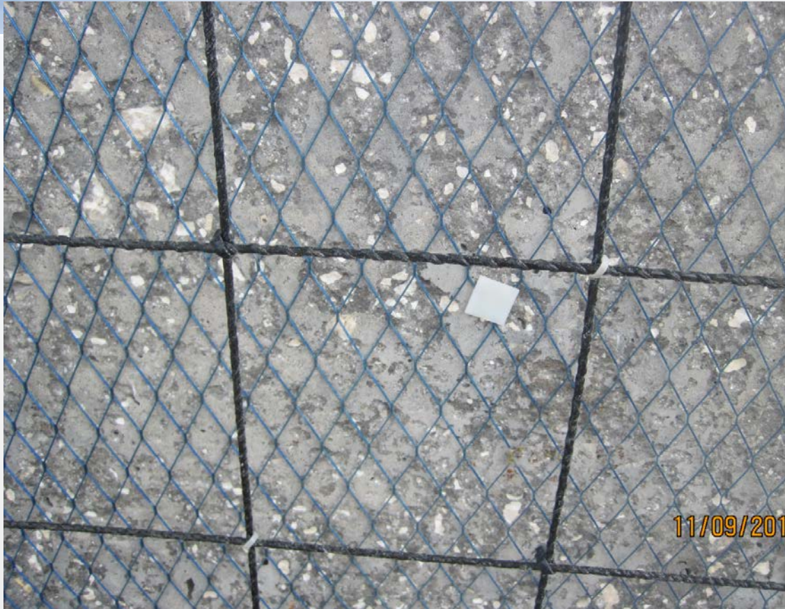
Ti Mesh anode w/basalt reinforcement.
