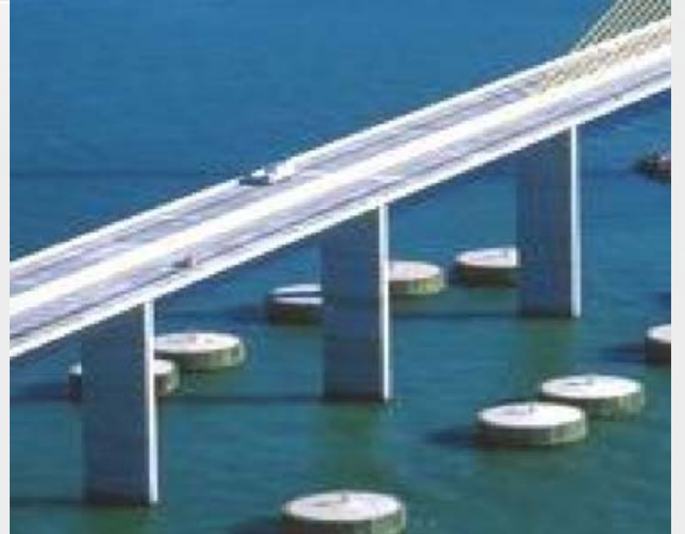
Main Span Columns (Impressed Current System)
