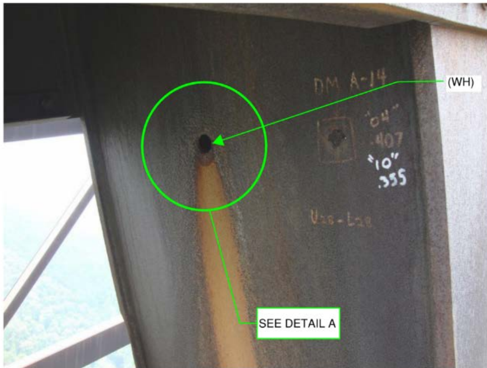
TYPICAL UPPER ARCH WEEPHOLE
