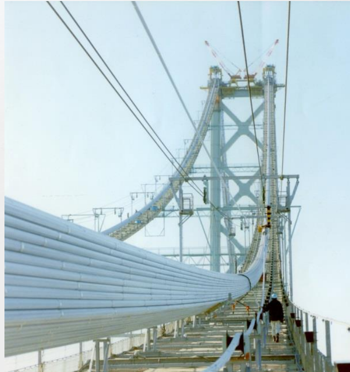
Prefabricated Parallel Wire Strand (PPWS)
