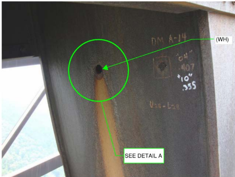
TYPICAL UPPER ARCH WEEPHOLE
