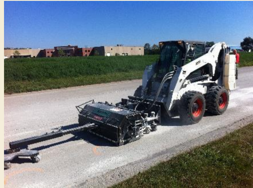
Bump Grinding on Surface Course
