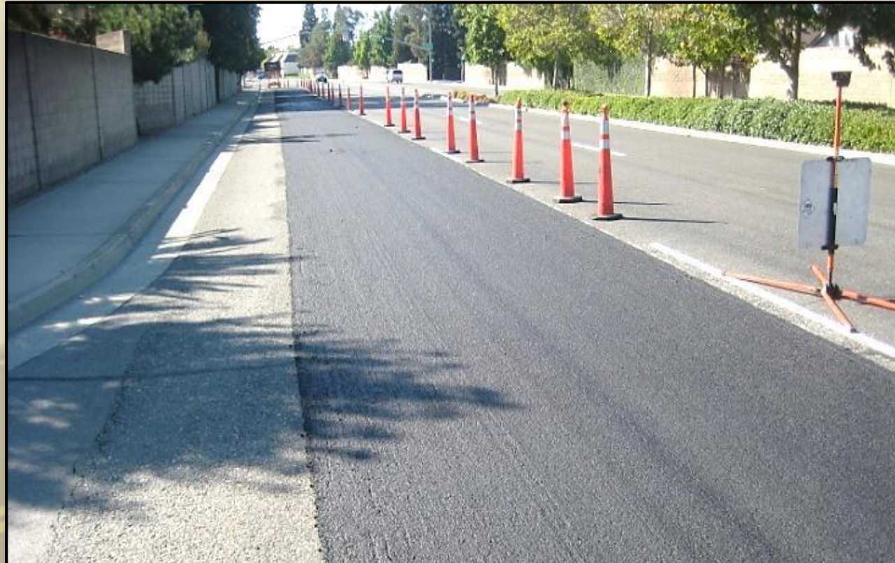
Microsurfacing on Arterial Street Cost: $ .39 per Square Foot
