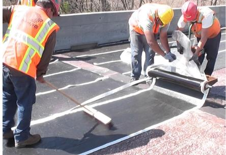
Deck Overlays – Fabric Membrane, Option 2 2-ply fabric w/ PG Binder
