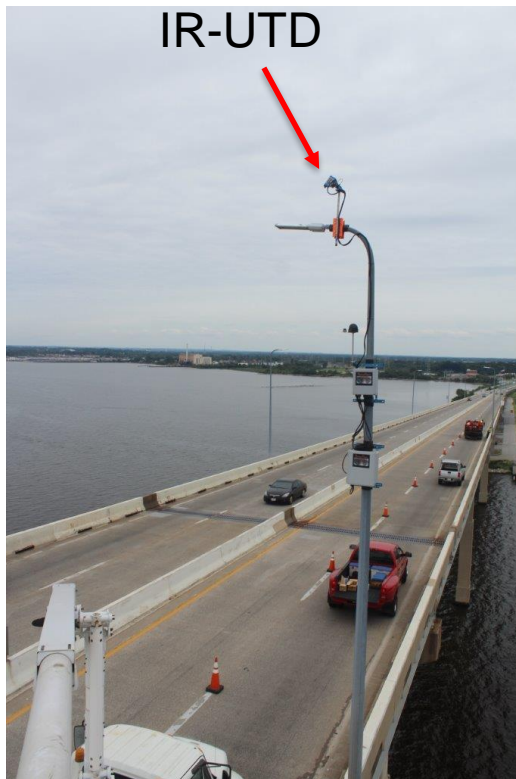
Existing light pole
