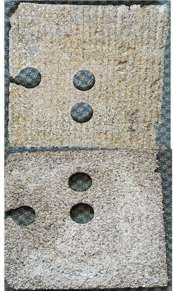
Delaminated overlay from a S8 specimen
