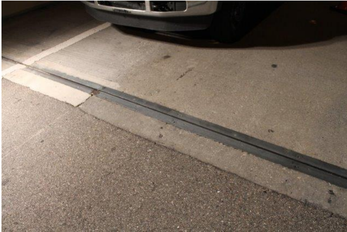
Armored Joint Repairs
