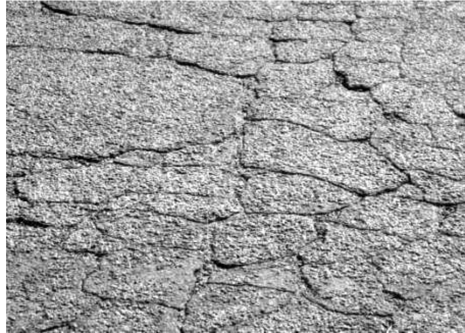
Block Cracking
